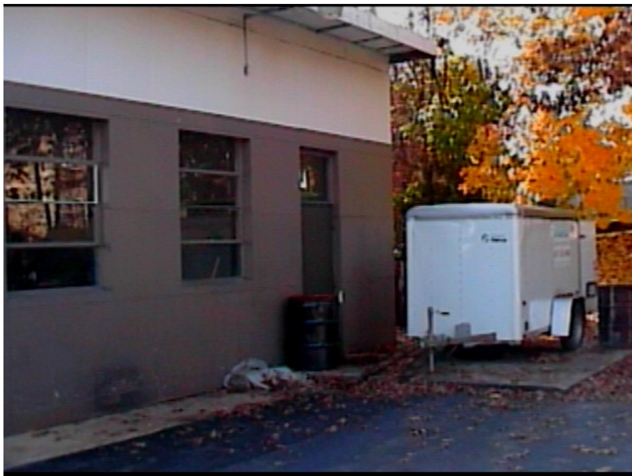
Photo 2: Small Trailer-Mounted System at Ron Moyer Service Center
