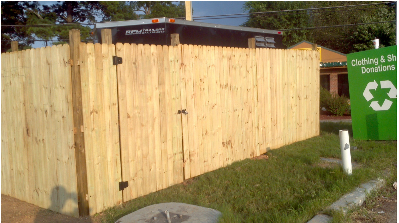
System in Fence Enclosure
